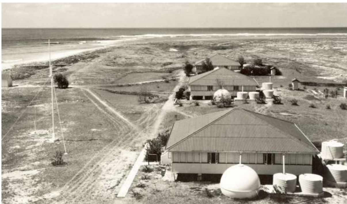
Figure 4. Lady Elliot Island cottages, undated (Source: Australian Maritime Safety Authority)
