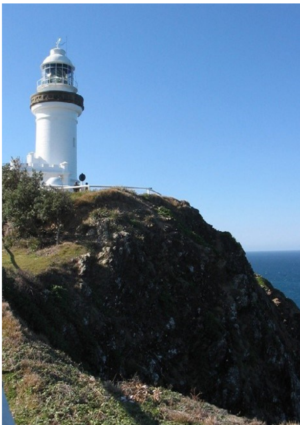
Figure 5. View of Cape Byron Lighthouse and surrounding cliffs (2005)
