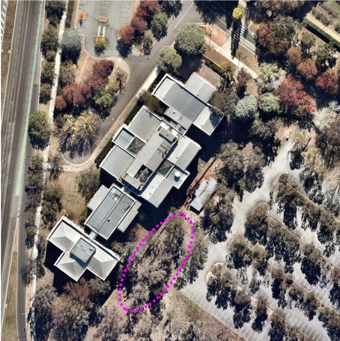
Figure 51 Aerial view of West Block: the location of an indicative building envelope is in pink Source: www.nearmap.com
