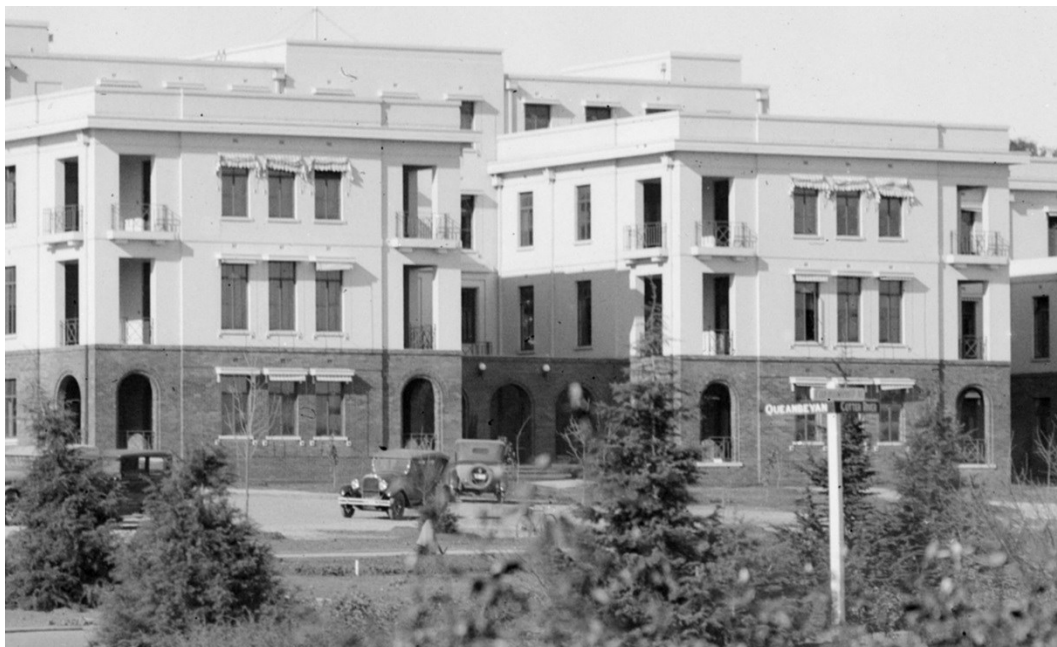
Figure 49 West elevation of West Block (part), c. 1928: the pull-down awnings in boxed casings were an early addition Source: National Archives of Australia, NAA A3560, 4323
