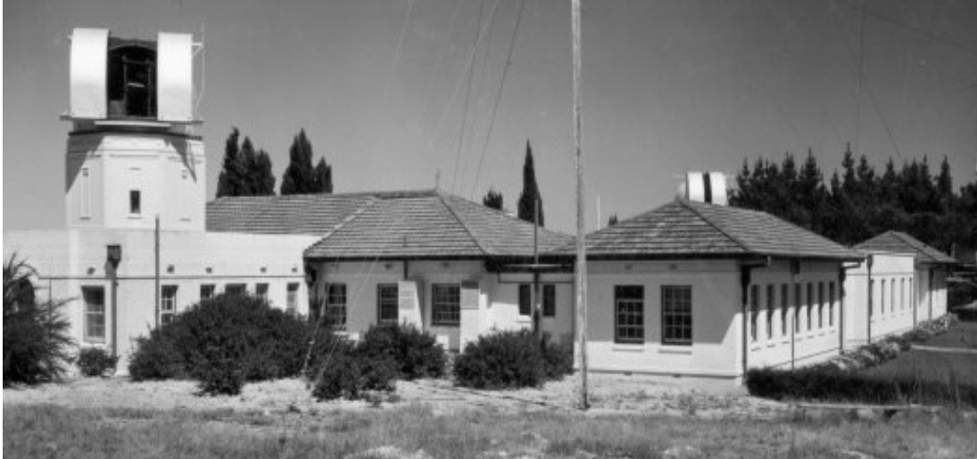
Figure 40 Mount Stromlo Observatory, established 1924 Source: ACT Heritage Library
