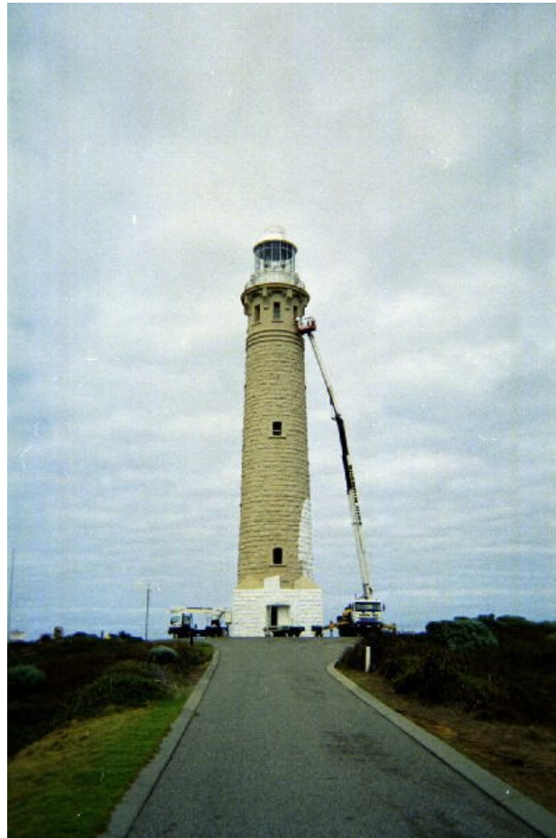
Figure 16. Repainting Cape Leeuwin Lighthouse (© AMSA, 2002)
