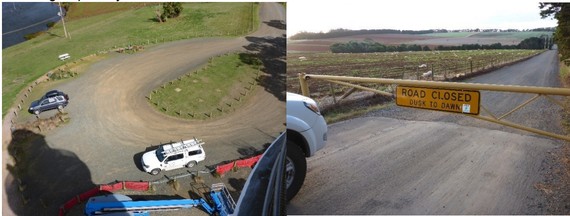
Figure 8. Roundabout and carpark at base of lighthouse tower (© AMSA, 2018).
