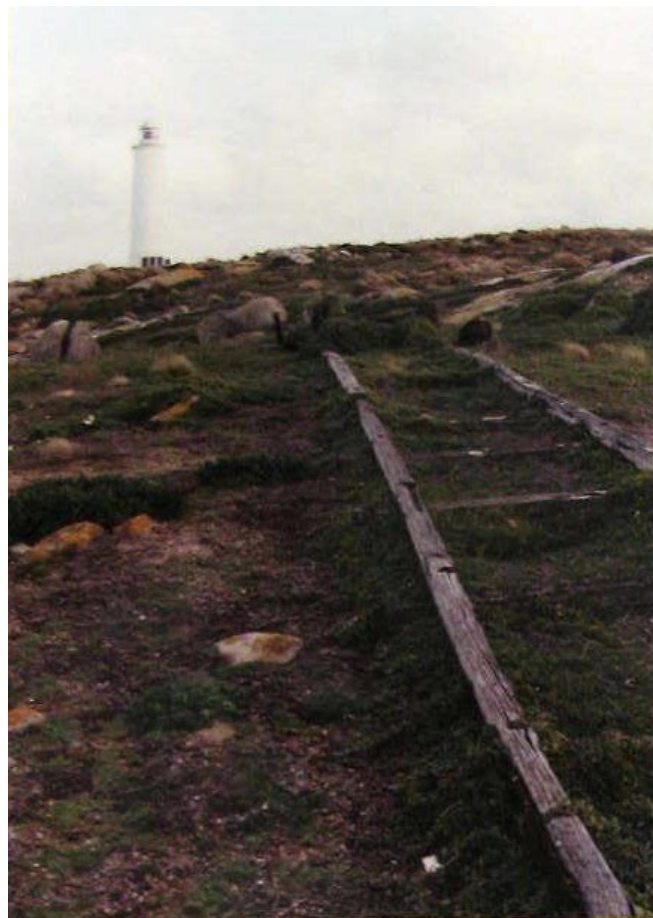
Figure 13. Goose Island tramway, 1990. Image courtesy of the National Archives of Australia: P2812, 18 (© Commonwealth of Australia, National Archives of Australia)
