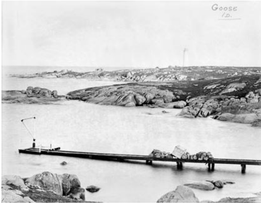
Figure 12. Goose Island jetty and tramway (1917). Courtesy of the National Archives of Australia. (© Commonwealth of Australia, National Archives of Australia)
