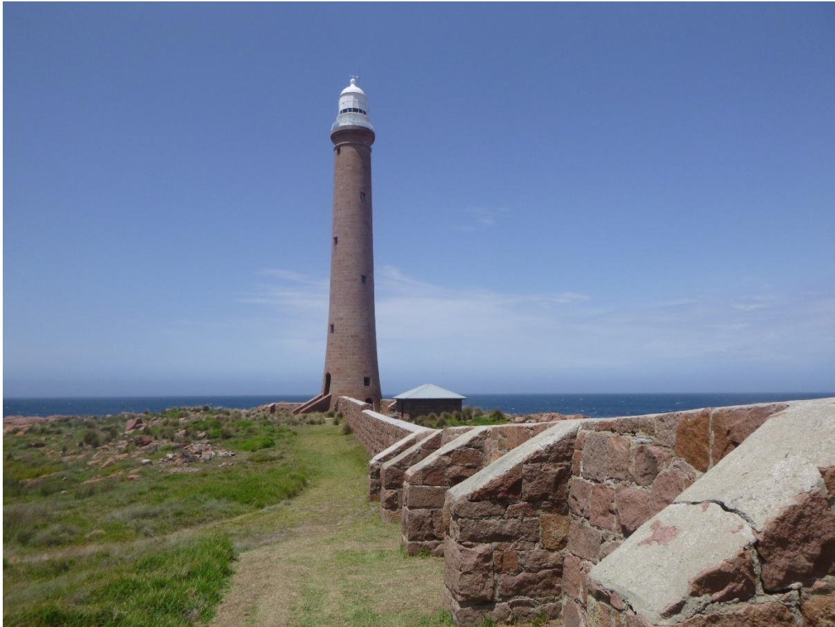
Figure 8. View of Gabo Island Lighthouse and windbreak wall (© AMSA, 2019)
