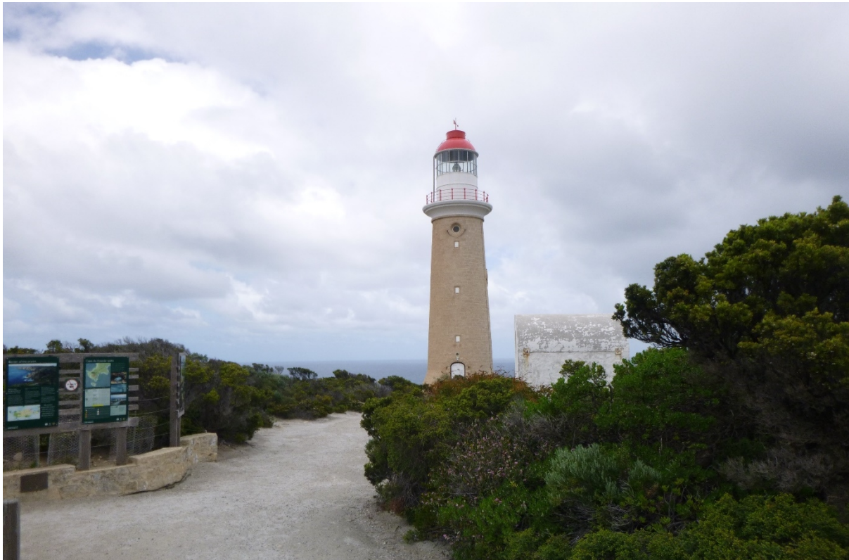
Figure 8. Access path to Cape du Couedic Lighthouse tower (© AMSA, 2021)
