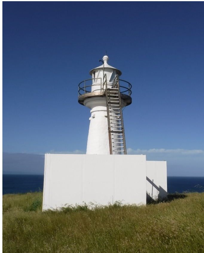
Figure 13. Cape St Albans tower with recent external ladder (© AMSA, 2017)
