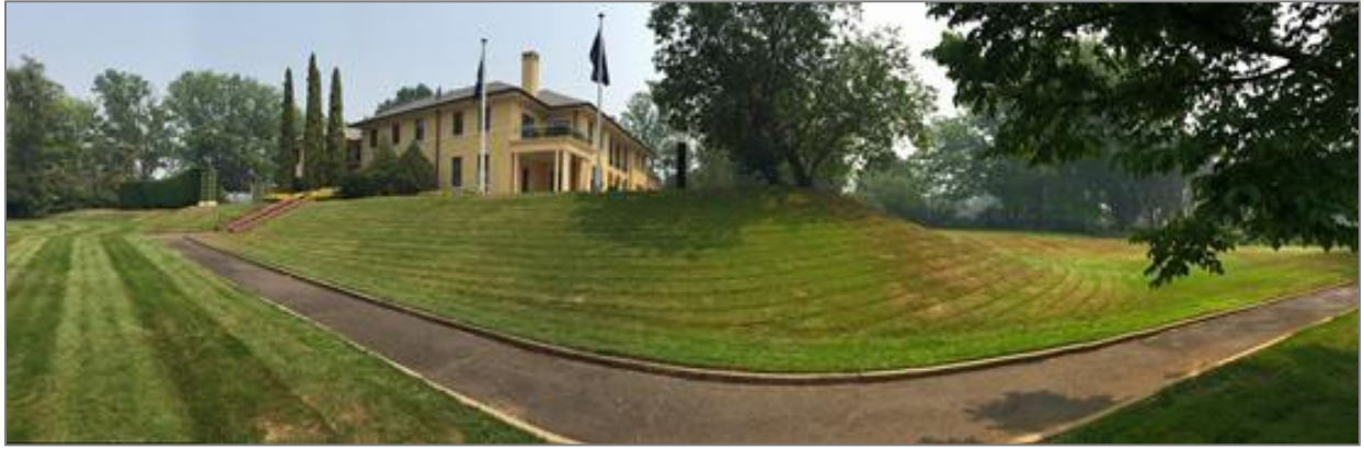
Figure 11: Panorama across the southeastern bank showing the precision of the original 1920s earthworks and the truncated path to the west. The southern lawn is to the left of the view.
