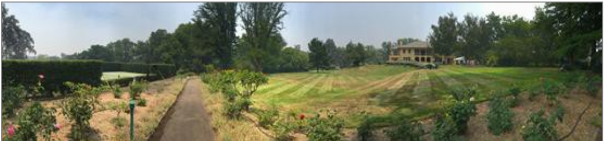
Figure 10: Panorama across the principal front space of The Lodge where the residence overlooks the drive loop, croquet lawn and tennis court. More recent intrusive actions include the awkward bedding in front of the building, cut-away sections of the original 1920s tennis court hedging and the security infrastructure.
