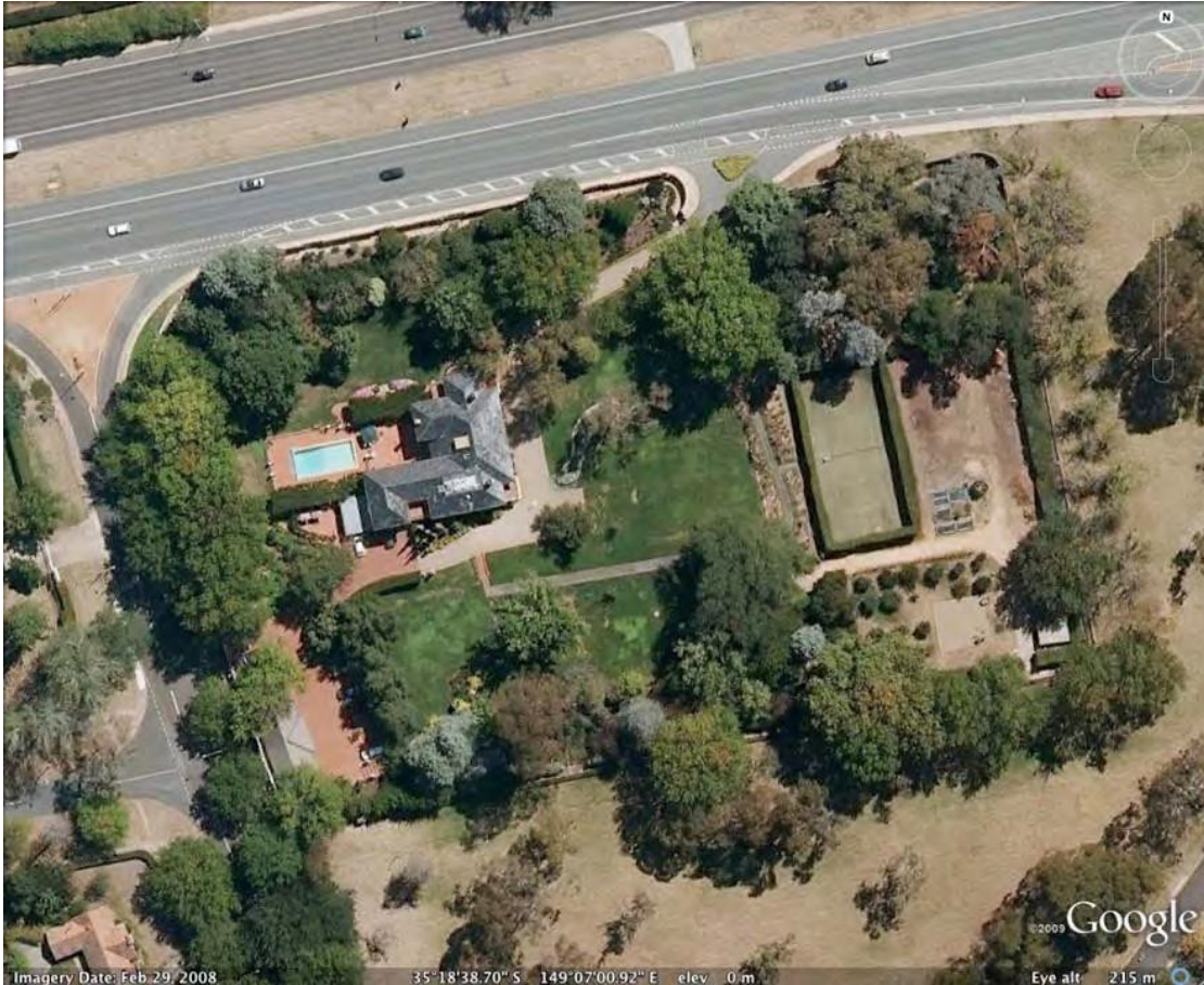
Figure 2: The Lodge (Google Earth image).
